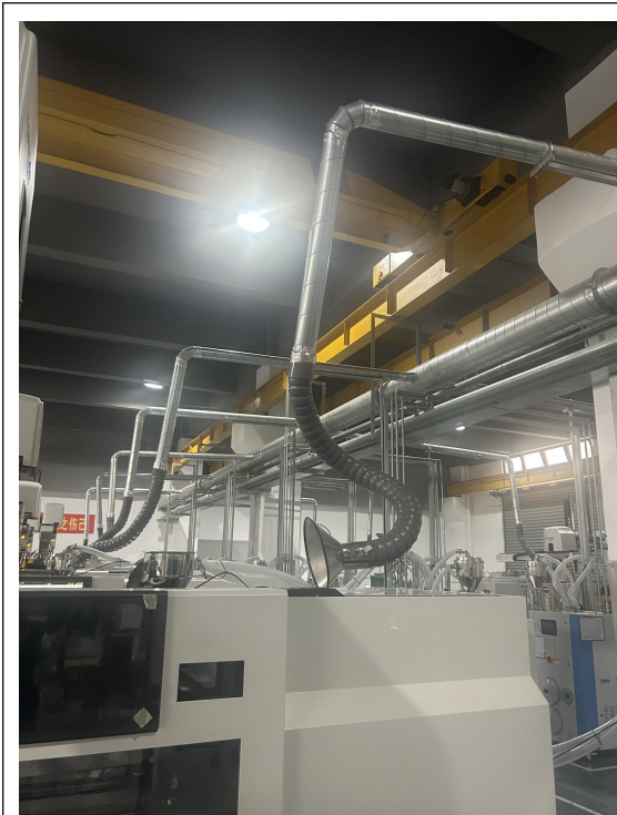
DA001 废气装置集气罩
